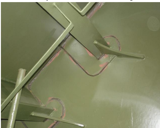
(c) Welds protected from coating for water tightness test
