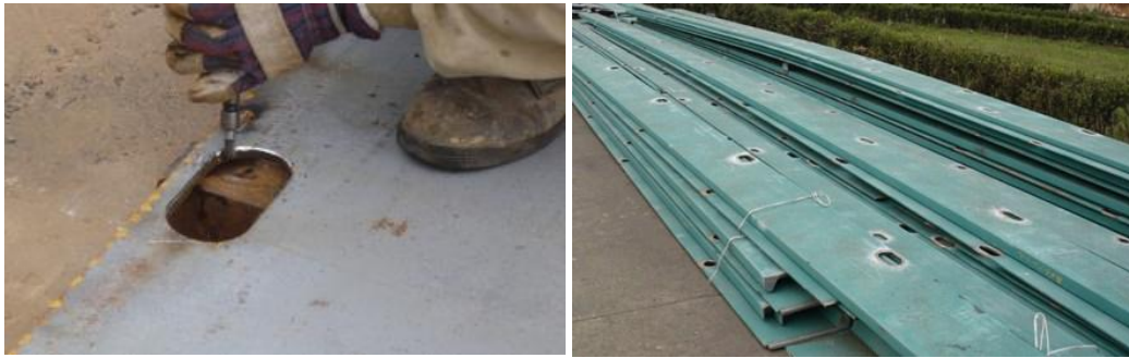
(a) Sharp edge grinding of all holes
