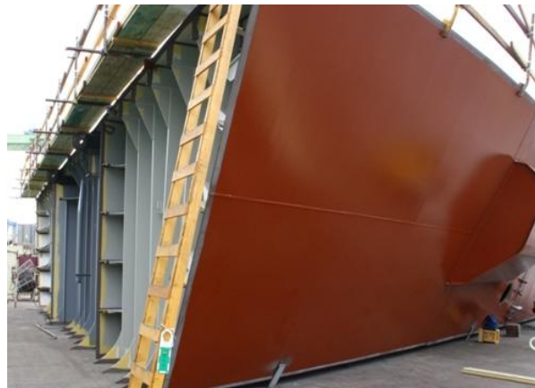
(b) The erection joint area is reduced dramatically after using masking tape.
