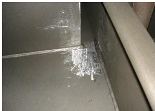
(d) Polished area by grinding
