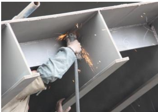
(c) Grinding after blasting is generally not permissible
