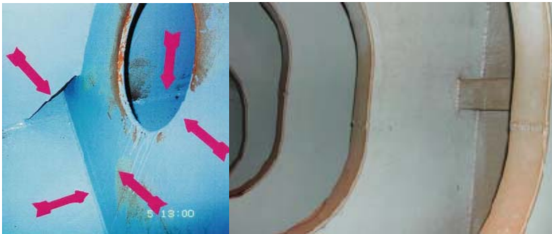
Figure 2 – Ultra High Solids Coating Performance After Three Years (left) and Eleven Years (right). At Three Years, Discoloration is Staining. At Eleven Years there is less than 1% Coating Damage
