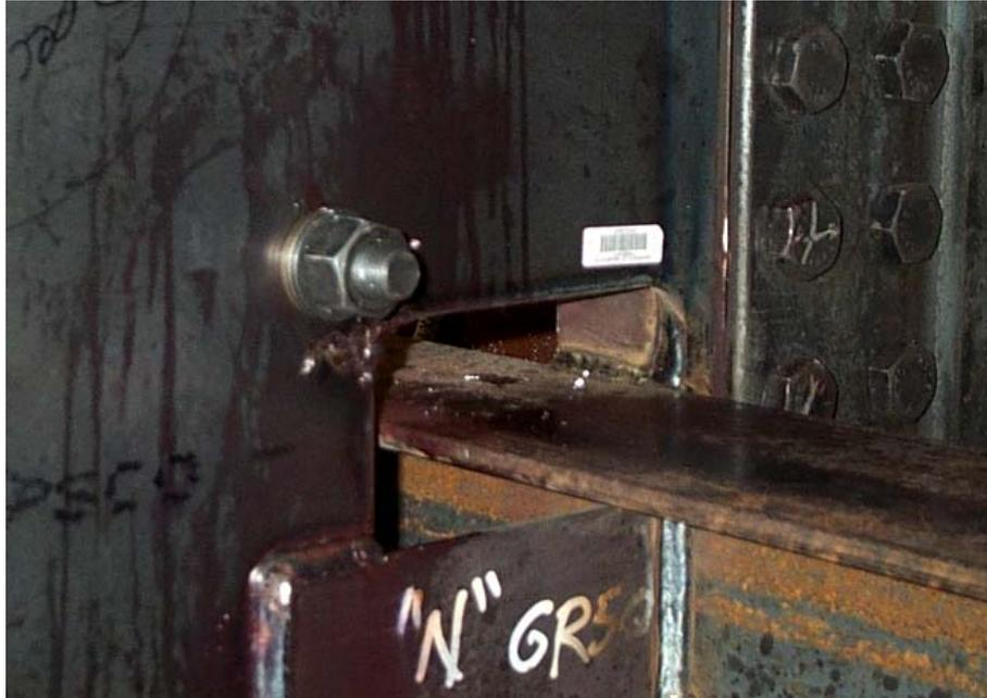
Figure 3.51 Repair of a crack in the web frame using a 24 mm stop hole and fully tensioned high-strength bolt
