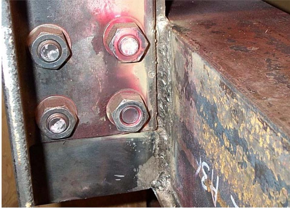
Figure 3.63 Weld repair at web frame-longitudinal connection
