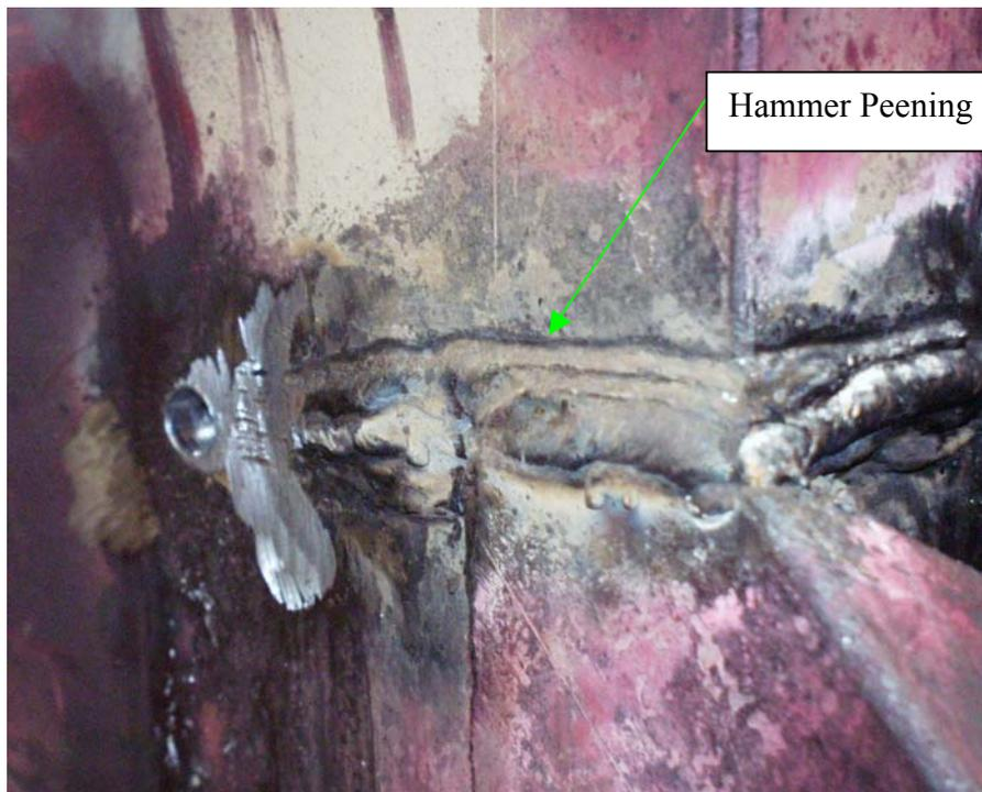
Figure 3.34: Weld that has been hammer peened after repair.
