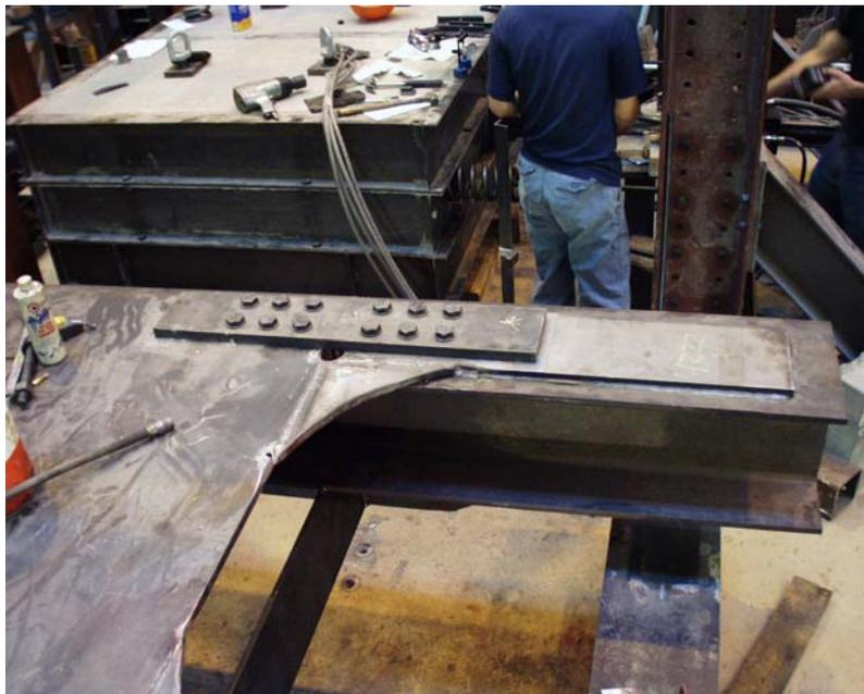
Figure 4: Bolted cover plate repair at a butt weld
