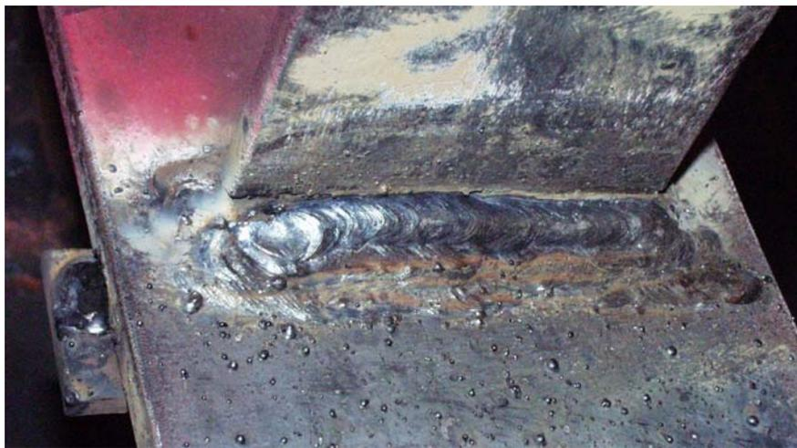
Figure 3.11: Single sided weld repair with backing bar.
