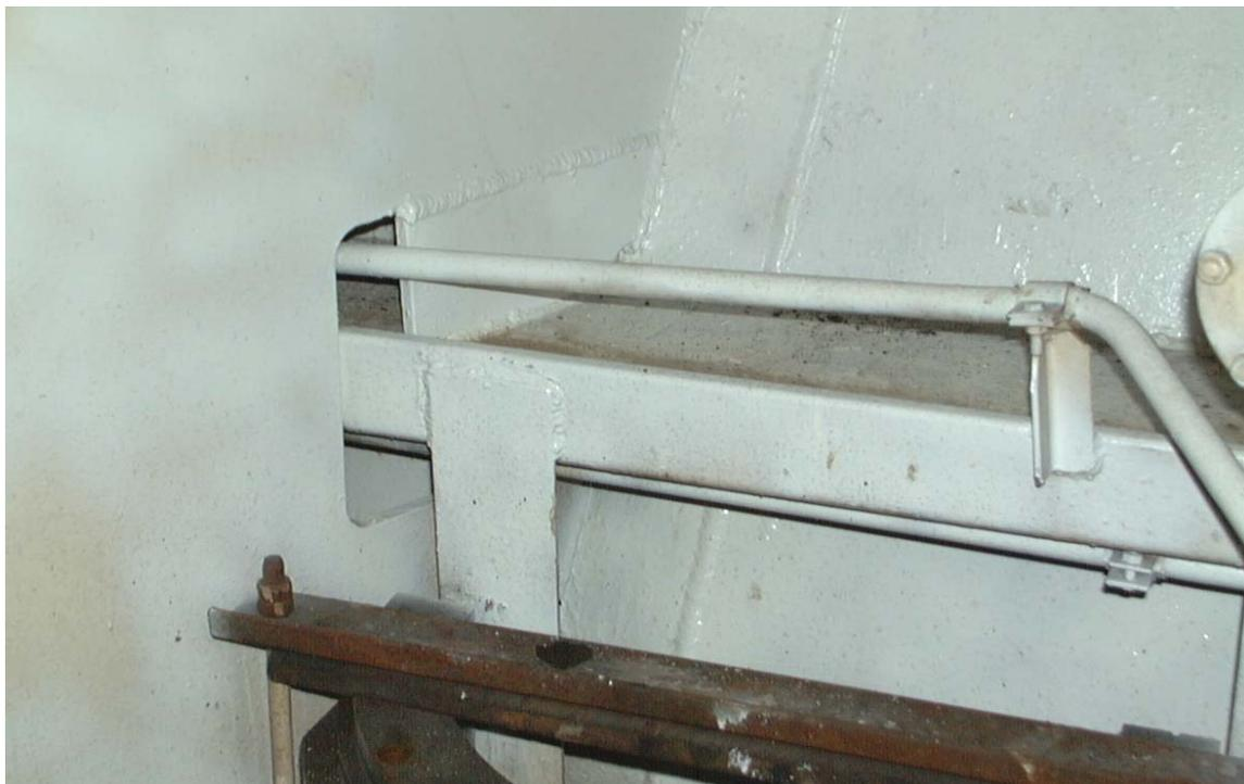
Figure 2.7: Longitudinal passing through a transverse web frame in a tanker ship [65]
