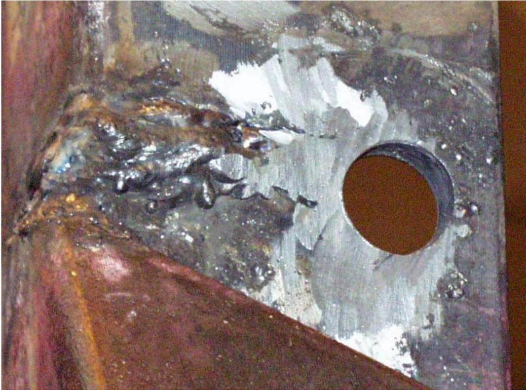
Figure 15: Weld repair of typical through-thickness crack with termination holes drilled to larger diameter after the weld is complete.
