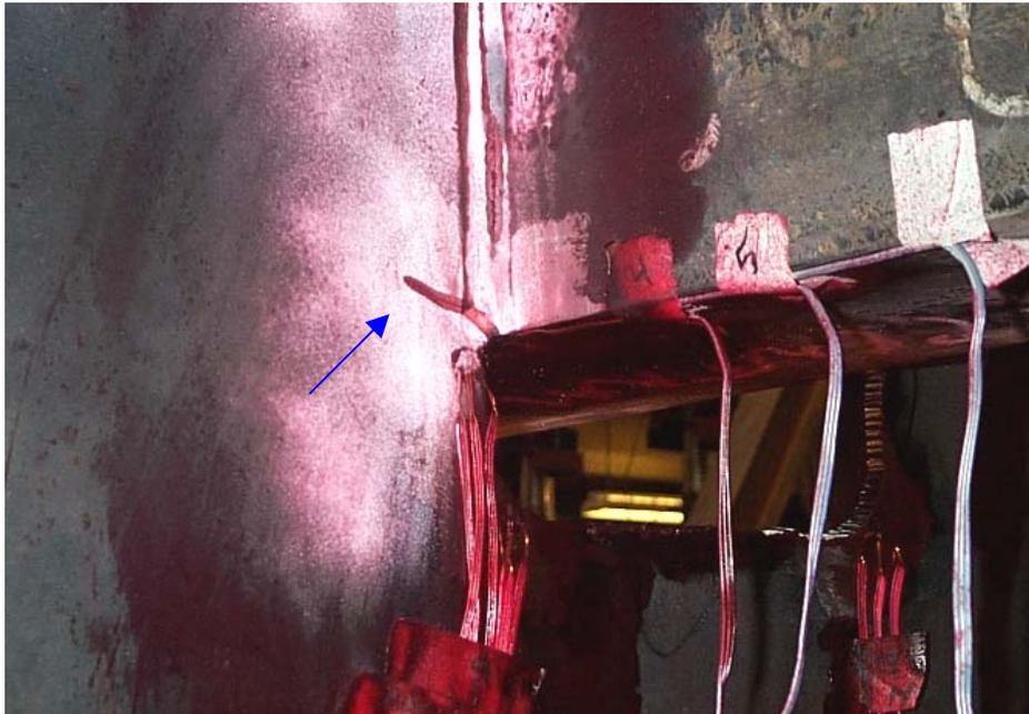
Figure 3.77: Typical crack in web frame at edge of longitudinal
