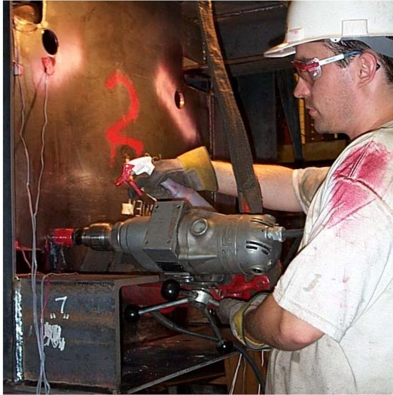
Figure 16: Drilling a stop hole using a magnetic base drill
