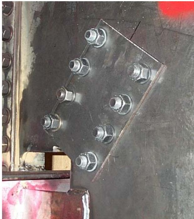
Figure 21: Bolted doubler plate
