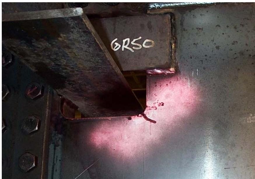
Figure 3.48 Typical crack in web frame growing out of a cutout
